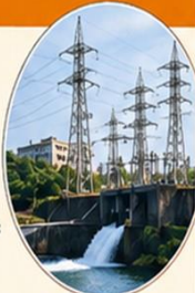
Hydroelectric Power Generation Center
